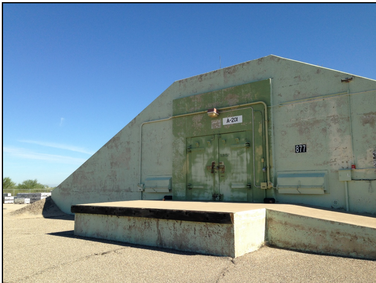
Figure 6-6. Steel door and reinforced concrete wall of Building 877.
