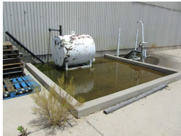
Photograph 28. Used oil AST in secondary containment outside the south wall of the Velocity Air south hangar. View to the northeast.
