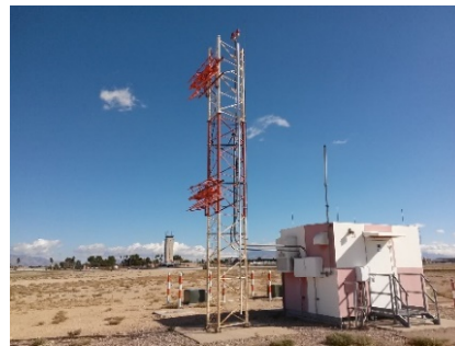
Example of a Localizer Antenna
