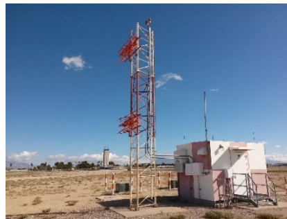
Example of a Localizer Antenna
