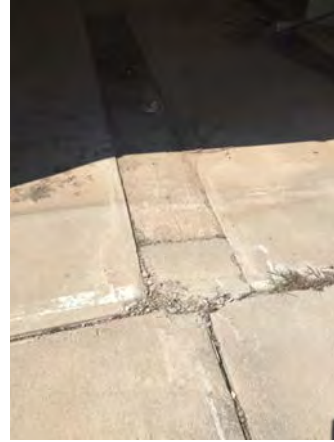
Photograph 44. Concrete-filled apparent linear drain in the center of the storage building. View to the northeast.
