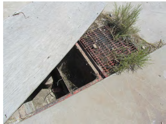
Photograph 36. Drain and separator in the wash rack pad.
