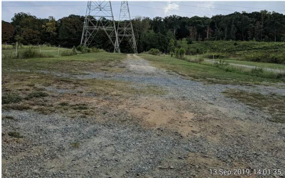
Photograph 1 – View of Site, Facing Northeast (dated September 13, 2019).
