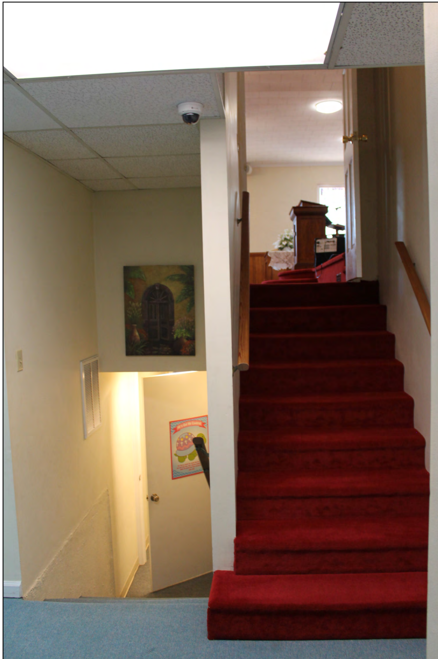
Figure 4.15: Sorrell's Grove Baptist Church (WA8802), stairs up from basement to addition and up from addition to sanctuary.
