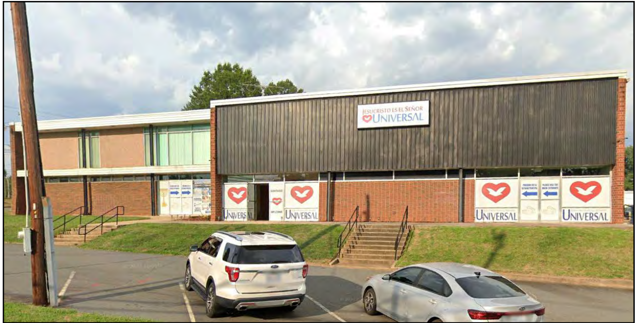
Figure 5.6: View of the Truck Drivers Union (AFL No. 71) Hall (Google Maps 2021).
