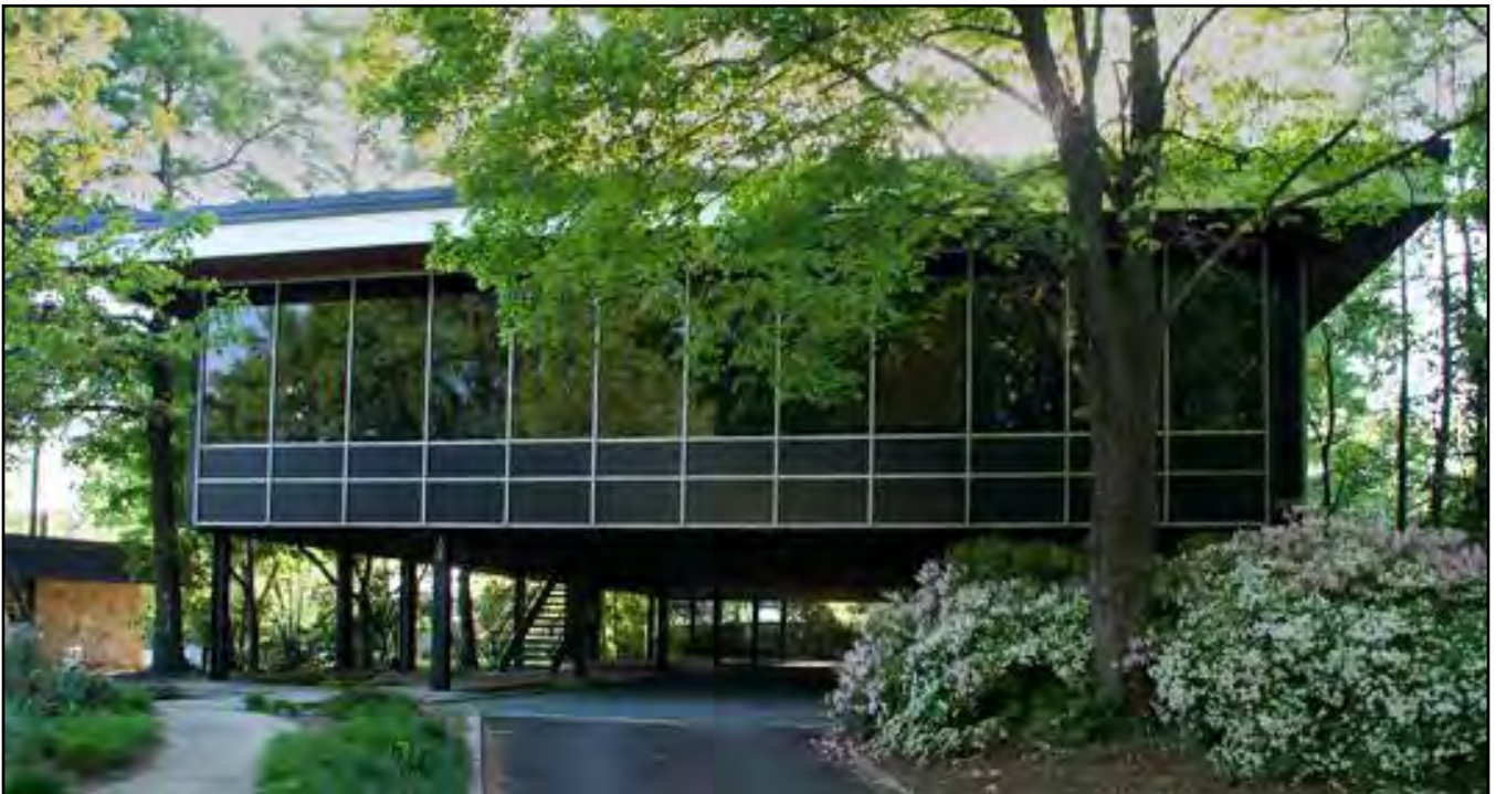
Figure 3.3: The G. Milton Small & Associates Office in Raleigh (Raleigh Historic Development Commission).
