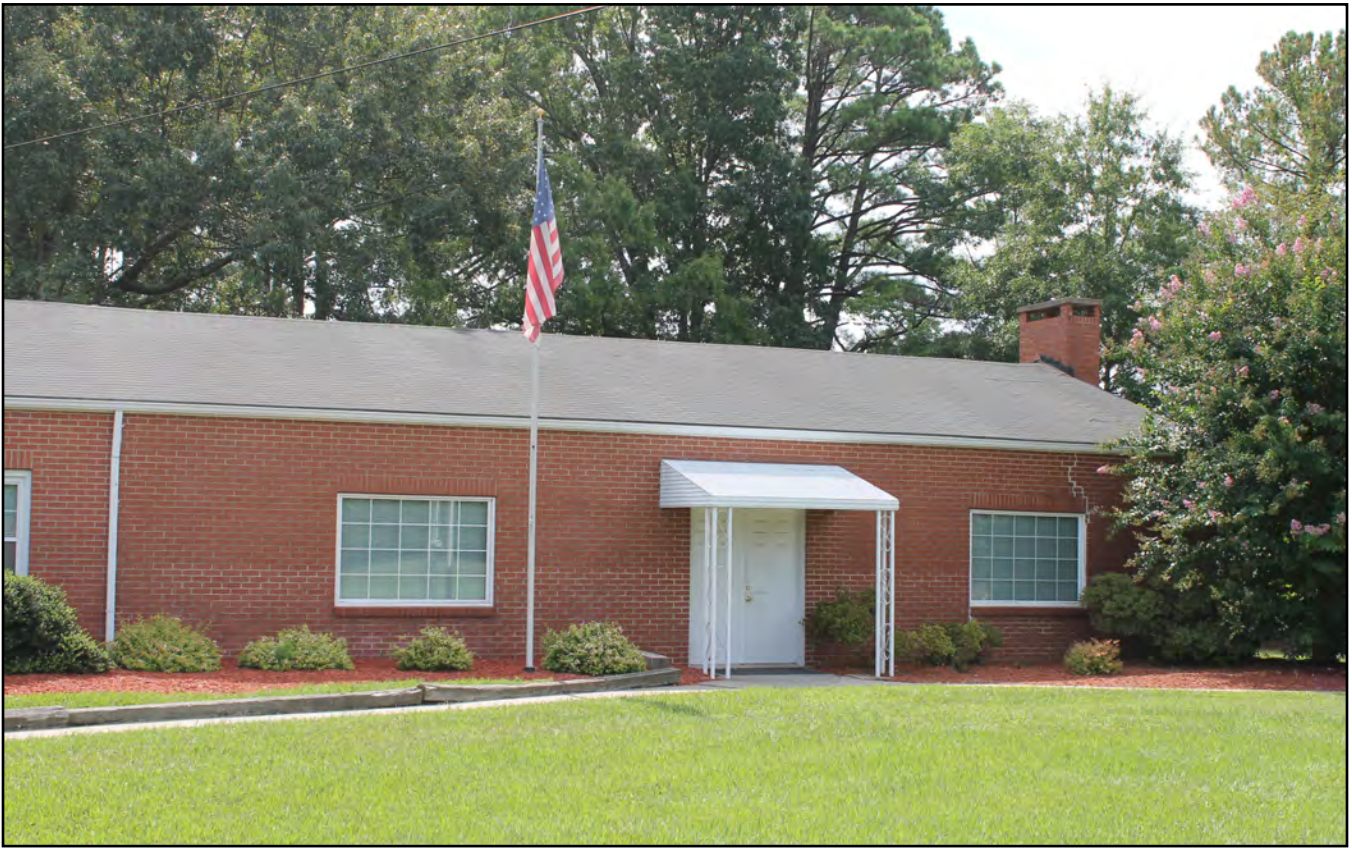
Figure 4.8: Sorrell's Grove Baptist Church (WA8802), fellowship hall, front (northwest) elevation.
