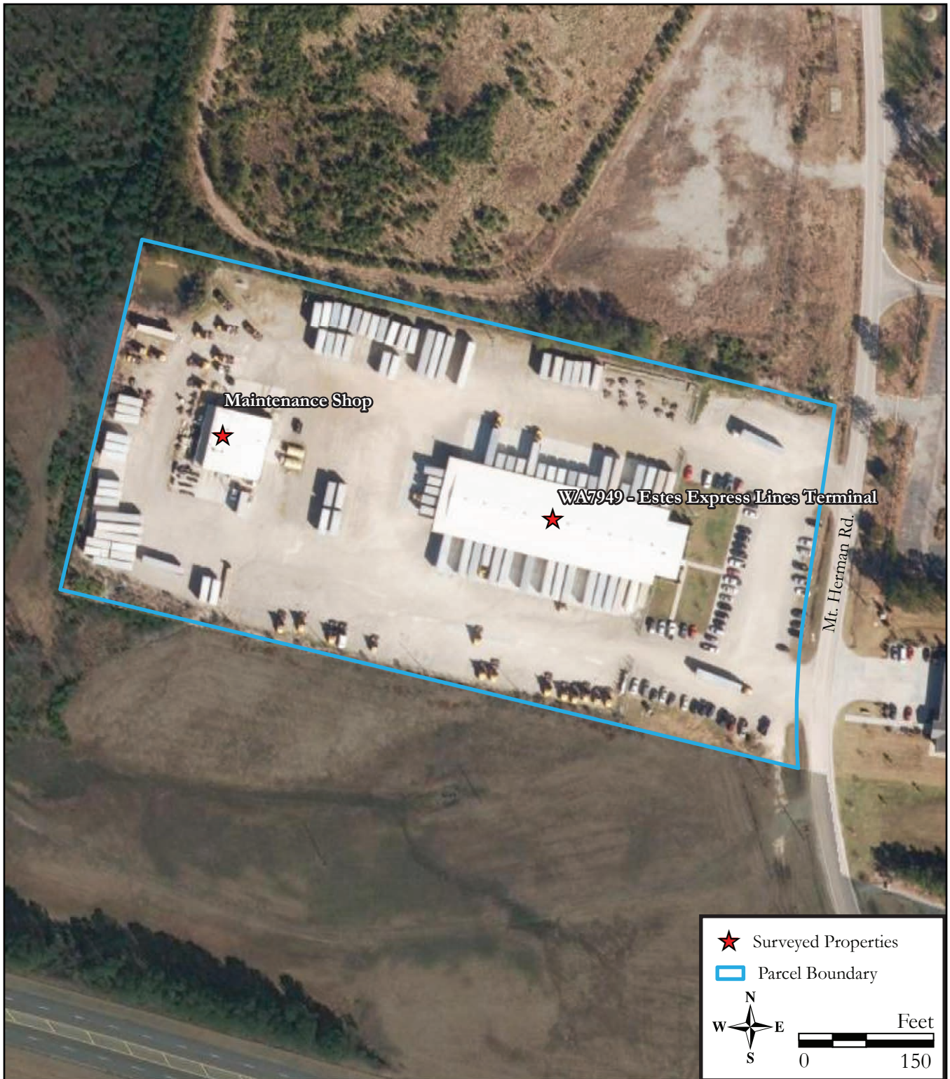
Figure 4.1: Aerial image of the Estes Express Lines Terminal (WA7949) (World Imagery, ESRI 2021).
