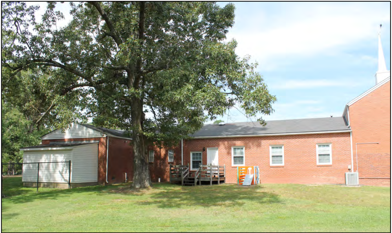
Figure 4.10: Sorrell's Grove Baptist Church (WA8802), fellowship hall wing rear (southeast) elevation.
