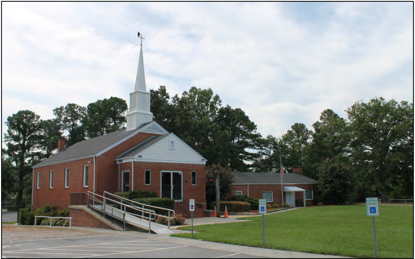
Figure 4.2: Sorrell's Grove Baptist Church (WA8802), overall view facing south.
