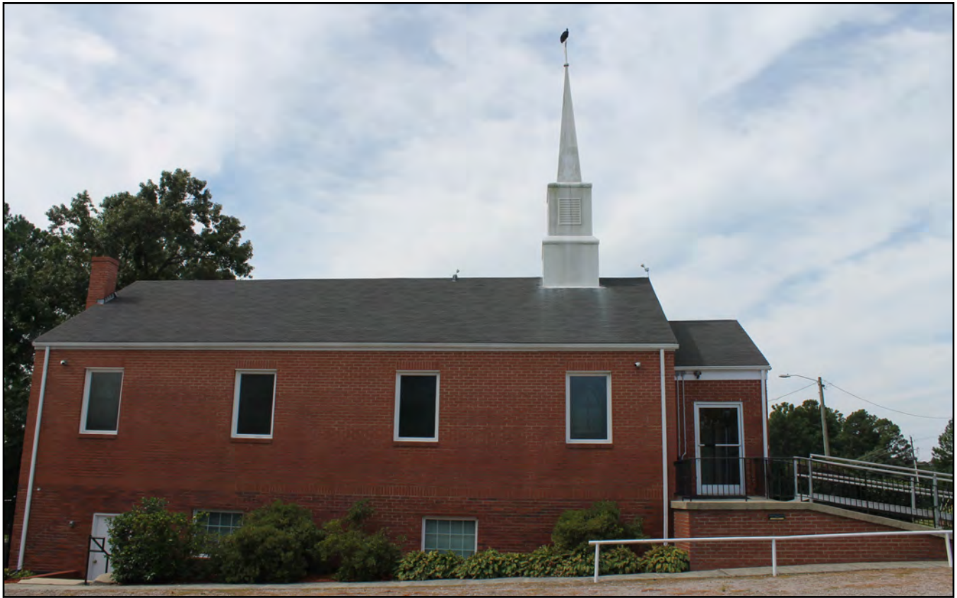
Figure 4.4: Sorrell's Grove Baptist Church (WA8802), northeast side elevation.
