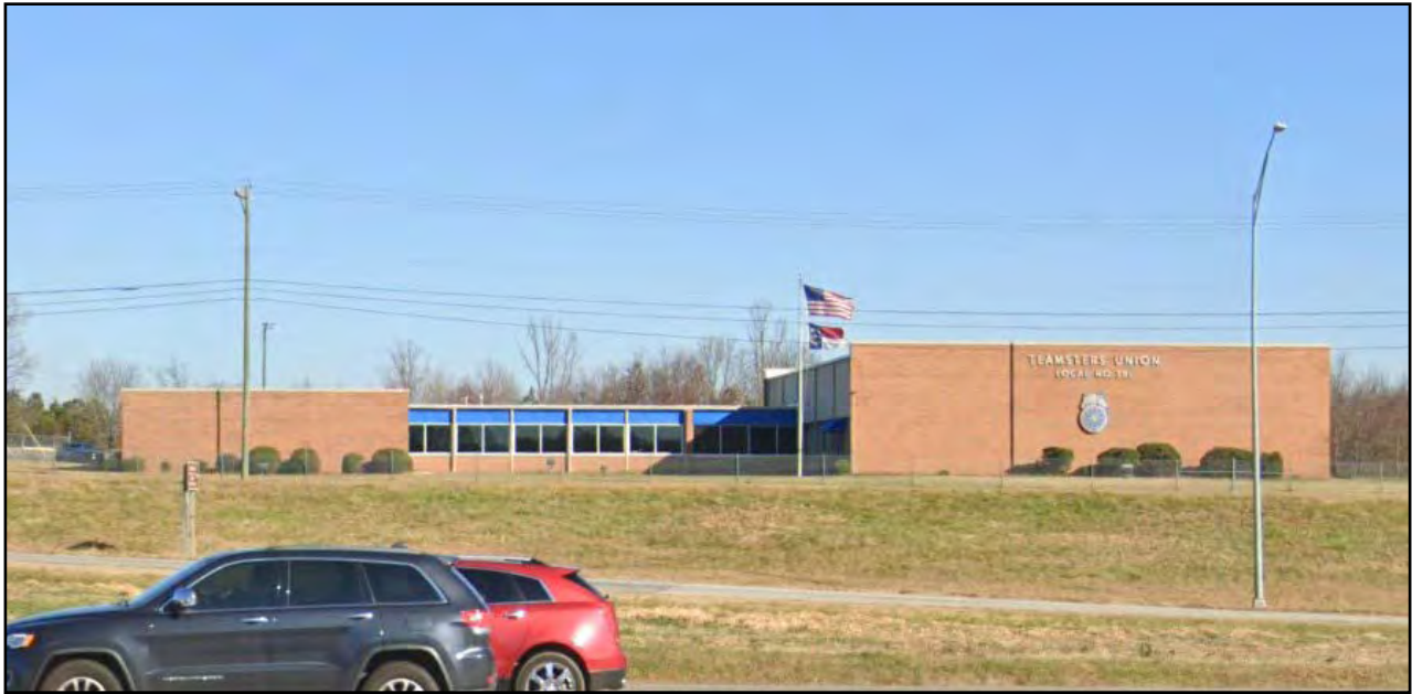
Figure 5.2: The Chauffeurs and Teamsters Union Local 391 Building (GF8970) in Colfax (Google Earth 2021).
