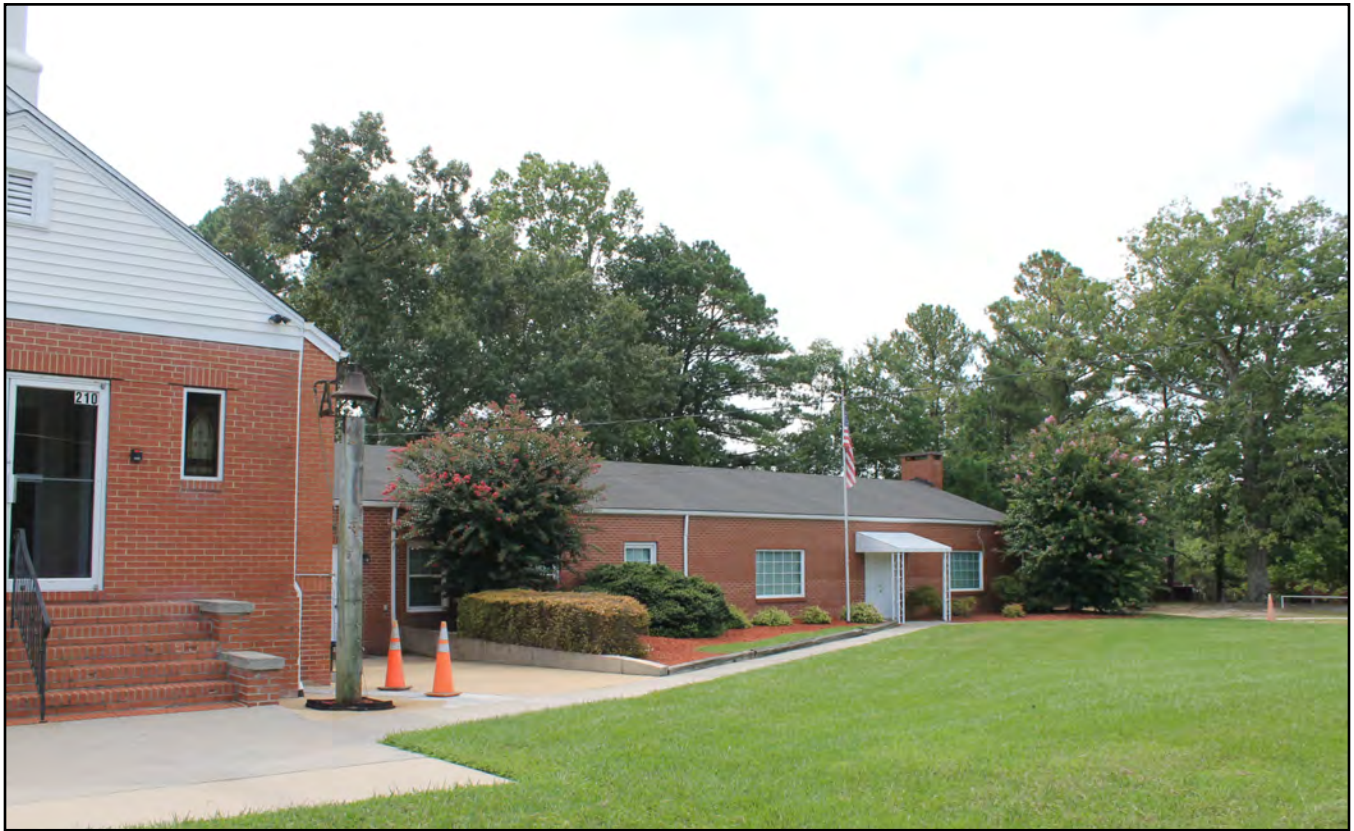
Figure 4.6: Sorrell's Grove Baptist Church (WA8802), fellowship hall wing, view facing south.
