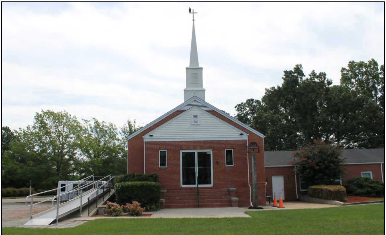
Figure 4.3: Sorrell's Grove Baptist Church (WA8802), front (northwest) elevation.
