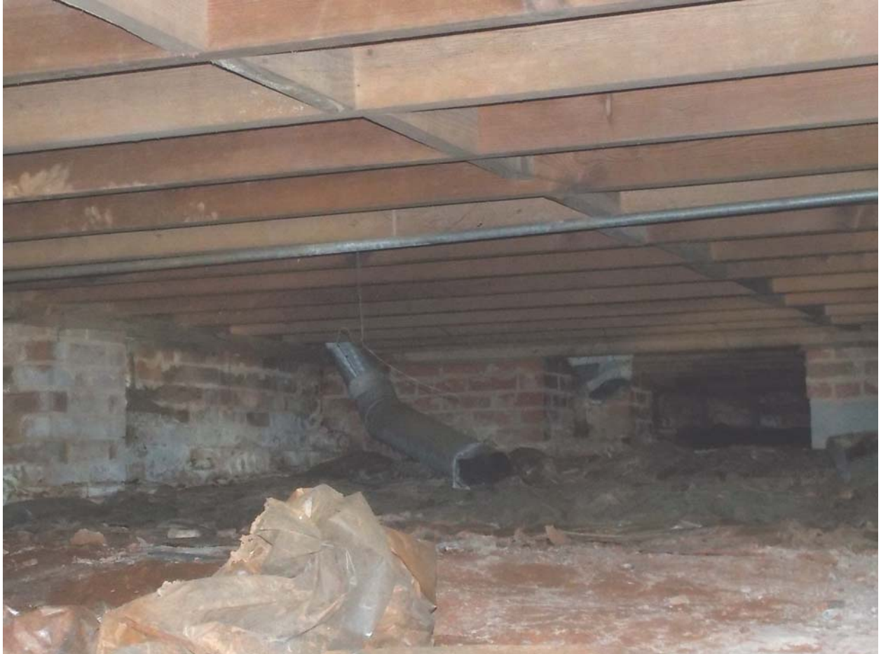
PHOTO 3 – WHITE HVAC DUCT JOINT WRAP – CRAWLSPACE
