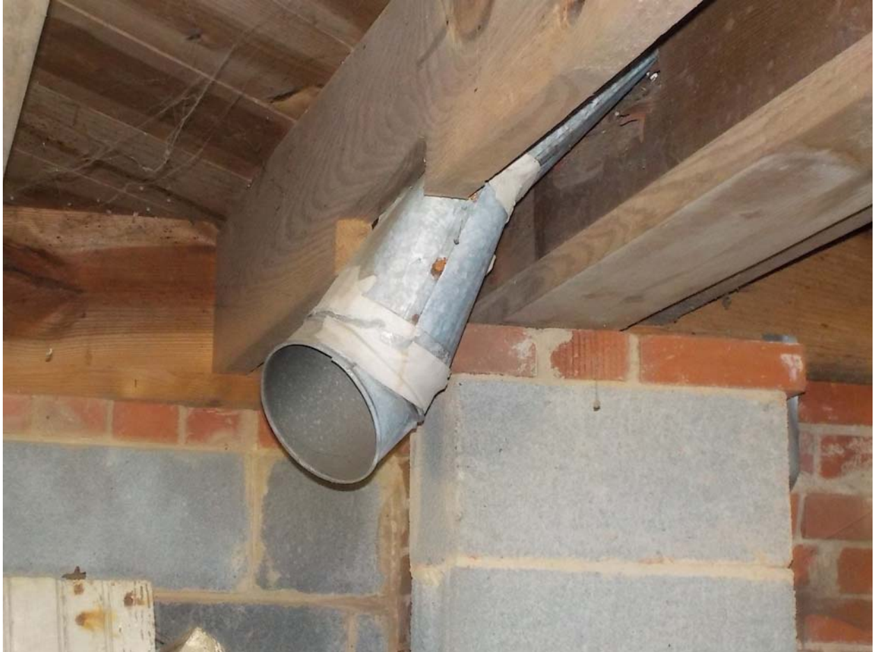
PHOTO 2 – WHITE HVAC DUCT JOINT WRAP – BASEMENT
