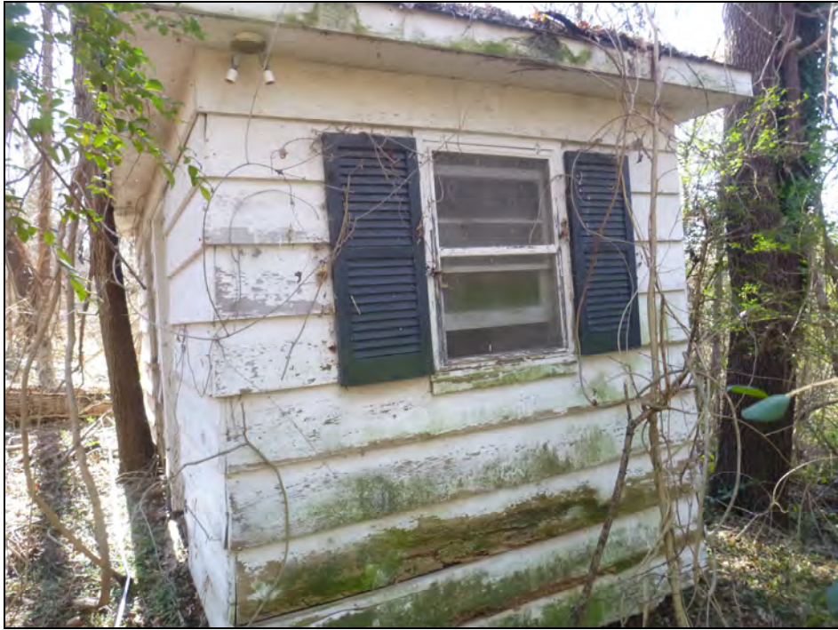
Figure 31. 31MK1151, Structure North Elevation, view south.
