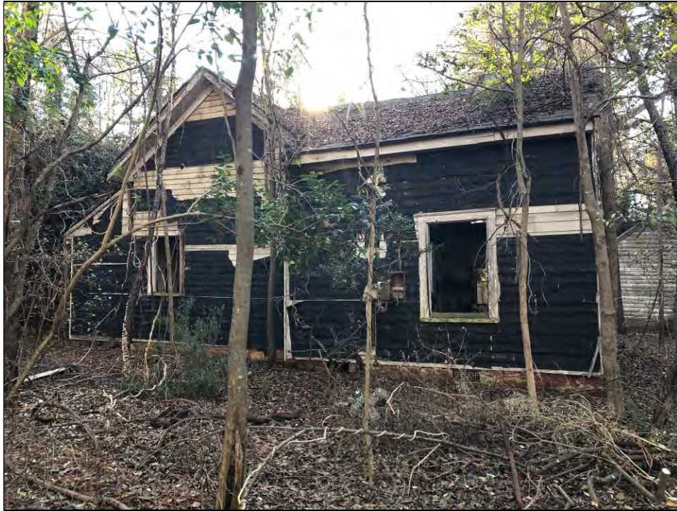
Figure 31. McGinn House (31MK1145) south elevation, view north (ESI December 19, 2018).
