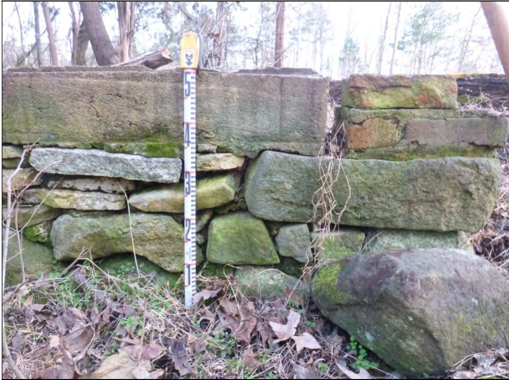
Figure 23. Site 31MK1144, close-up of stone-and-brick foundation, view northeast (ESI December 2018).
