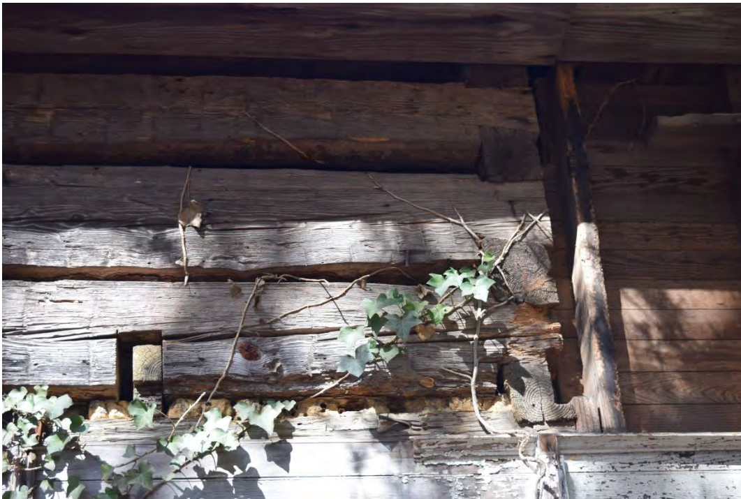
McGinn Family House, Façade, ca. 1855 Log Section, Detail of Log Notching.
