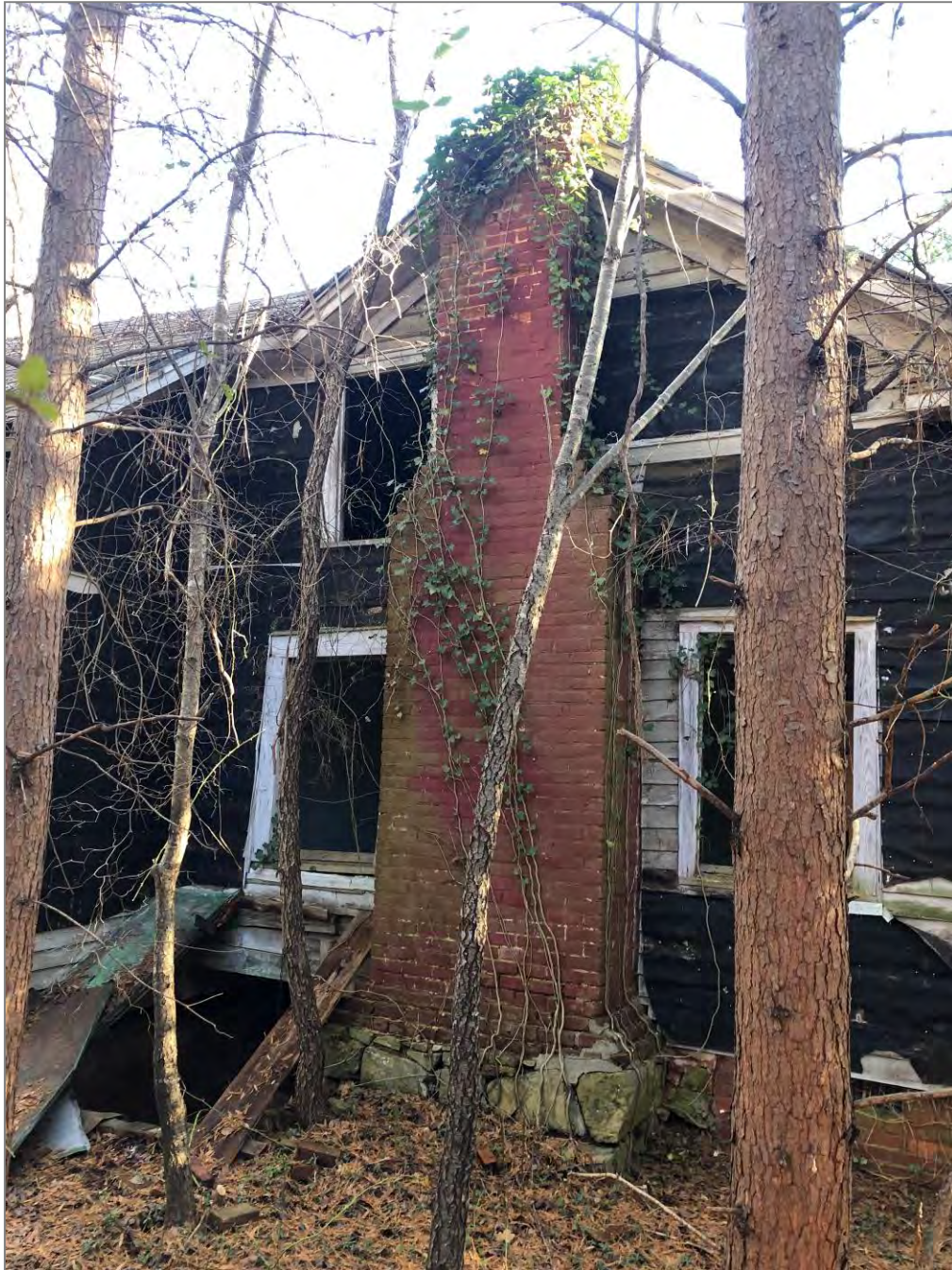
Figure 33. McGinn House (31MK1145) chimney west elevation (ESI December 19, 2018).
