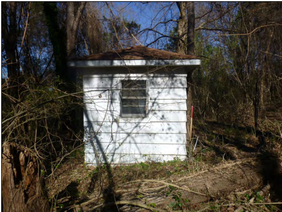
Figure 30. 31MK1151, Structure South Elevation, view north.
