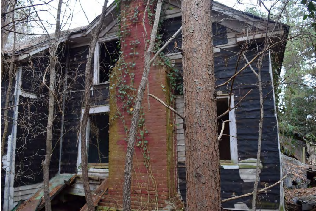
McGinn Family House, West Gable End and Chimney, ca. 1855 Log Section, Tar Papered Exterior, Looking East.
