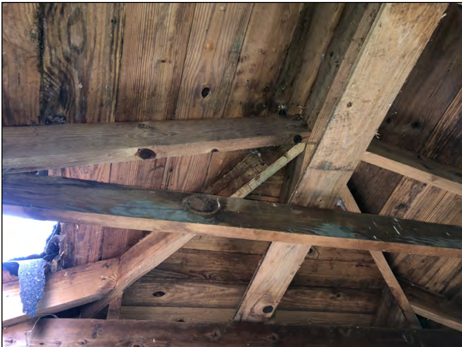
Figure 32. 31MK1151, Structure Interior Roof Framing.
