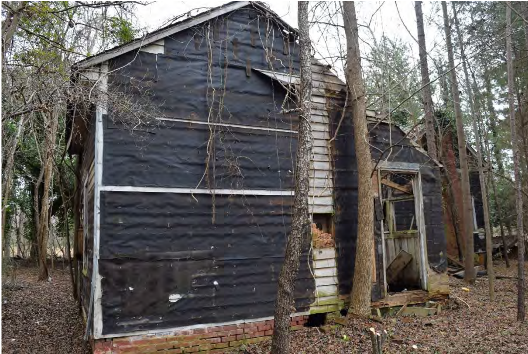
McGinn Family House, Rear Ell and Shed, West Gable End, Looking East.
