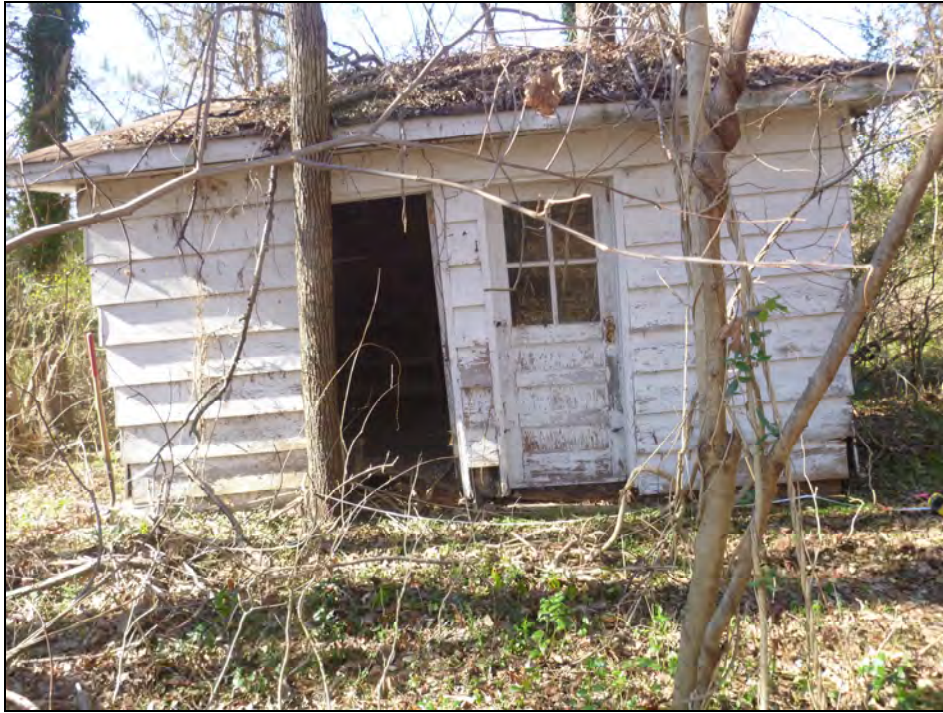
Figure 29. 31MK1151, Structure Exterior view west.
