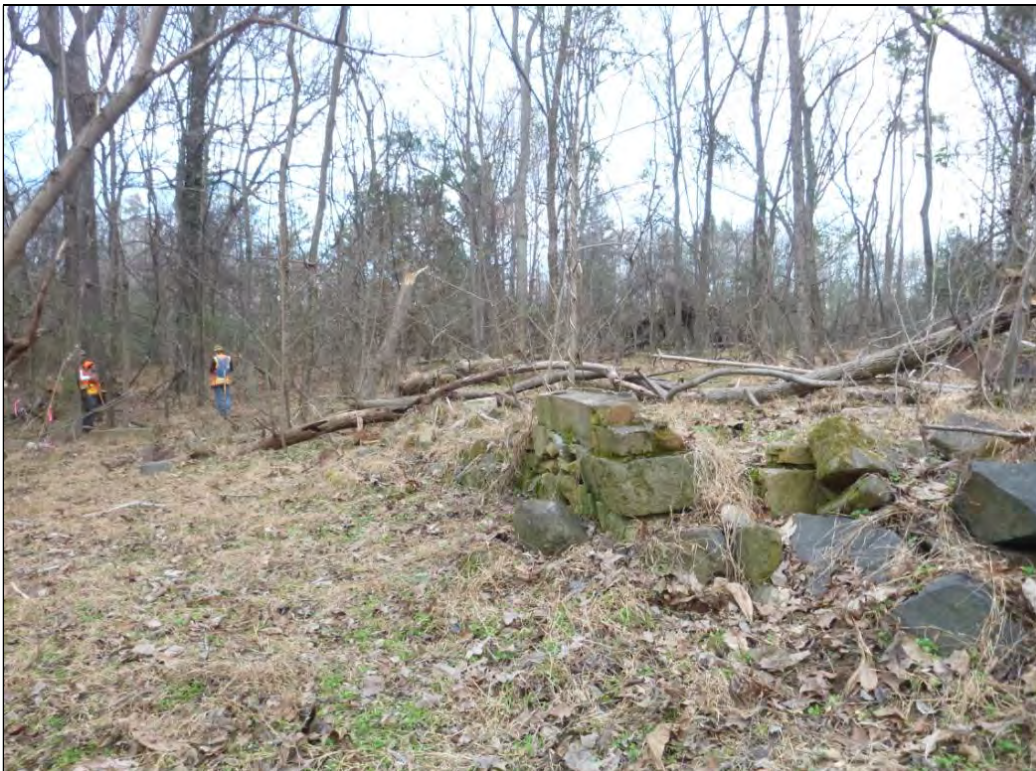
Figure 24. Site 31MK1144, overview of foundation, view northwest (ESI December 2018).
