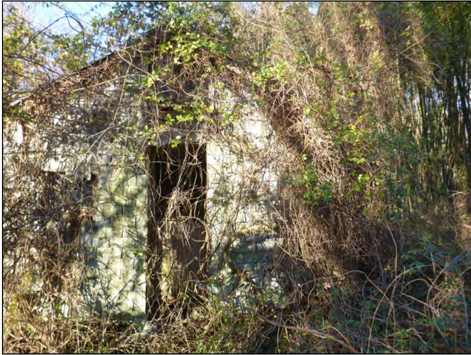
Figure 42. 31MK1154, structure near ST12-13, view west.
