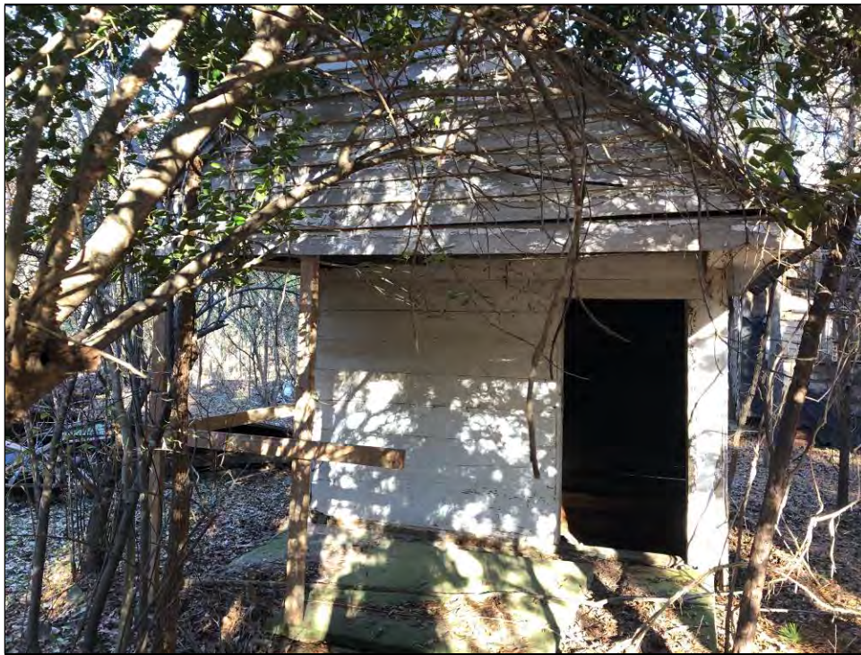
Figure 32. McGinn well house (31MK1145), view north (ESI December 19, 2018).
