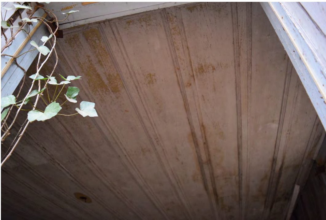
McGinn Family House, Interior, Board-and-Batten Ceiling, ca. 1855 Log Section.
