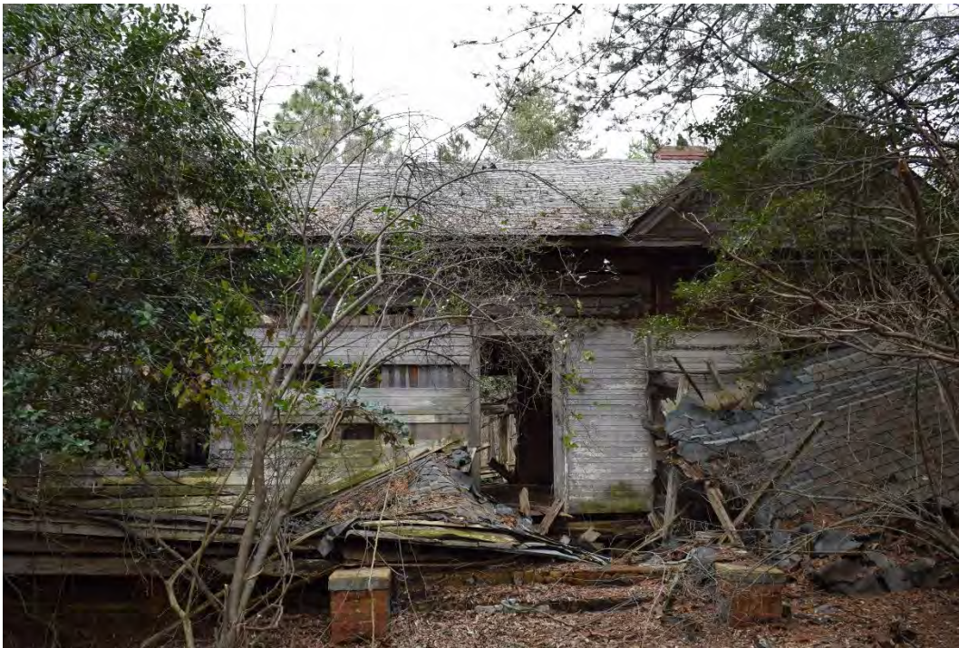
McGinn Family House, Facade, Looking North.
