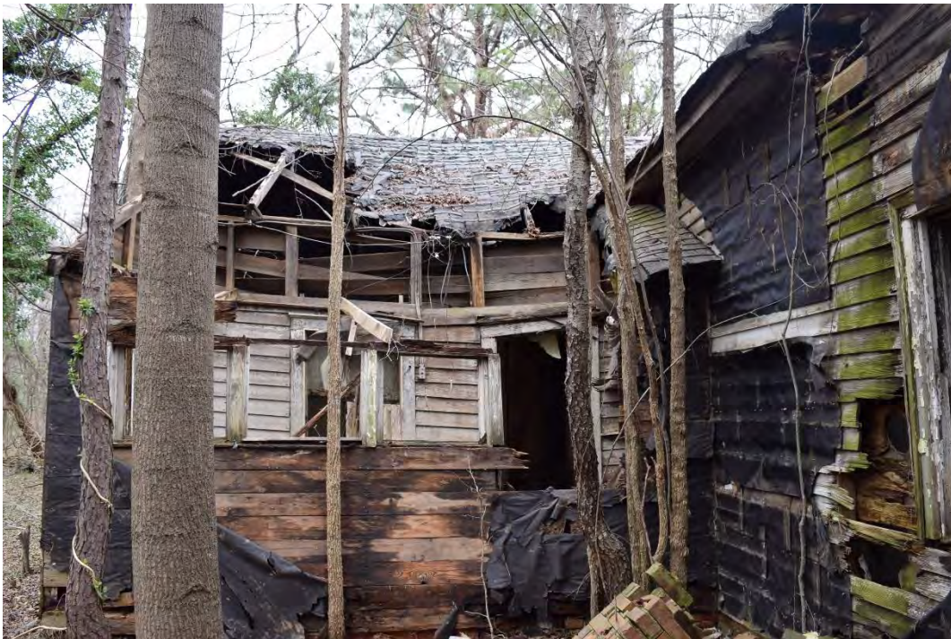
McGinn Family House, Rear Ell and Shed, Looking North.
