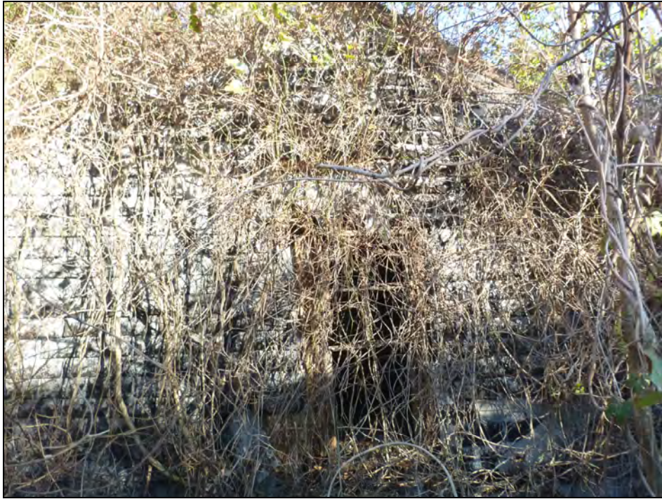
Figure 47. 31MK1154 structure, view east.
