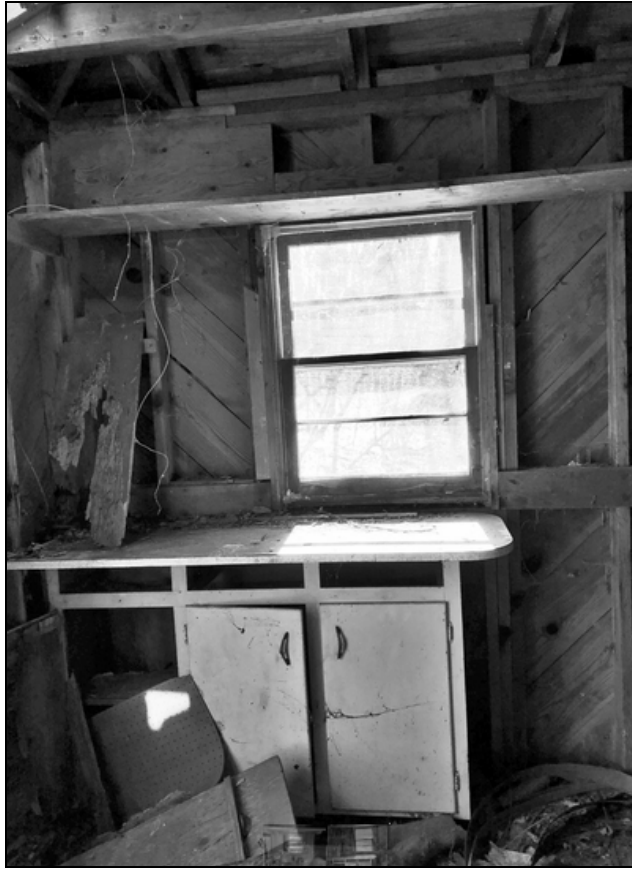
Figure 33. 31MK1151, Structure Interior South-Facing Wall.
