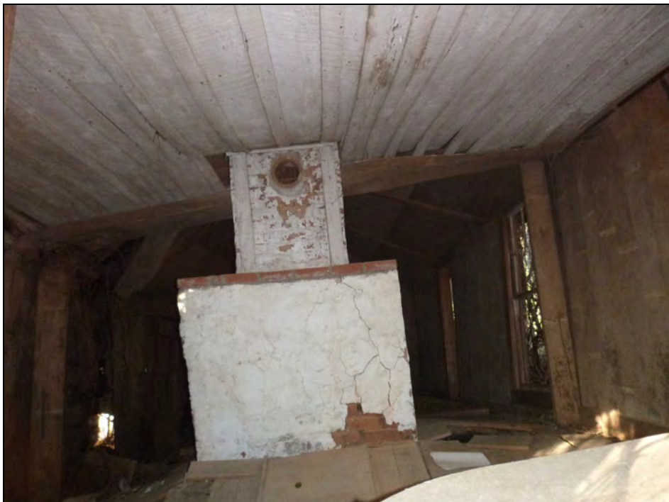
Figure 48. 31MK1154 interior, view west.
