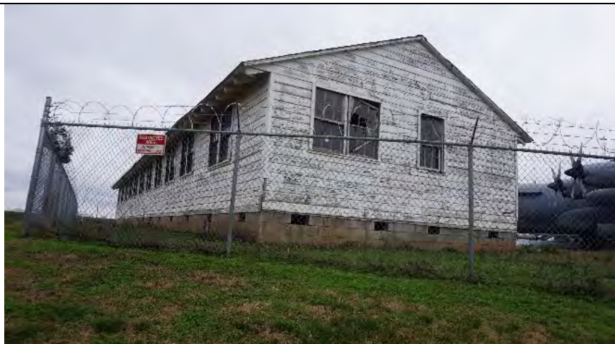
MK3825_ThomasW.FerebeeBuilding,ArmyAirCorpsMorrisFieldBarrac ks_02 20_V.W._03
