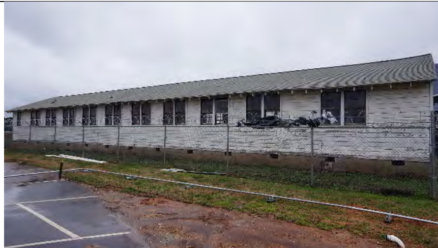
MK3825_ThomasW.FerebeeBuilding,ArmyAirCorpsMorrisFieldBarrac ks_02 20_V.W._02
