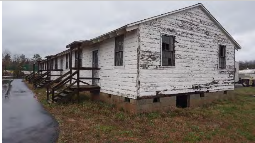
MK3825_ThomasW.FerebeeBuilding,ArmyAirCorpsMorrisFieldBarrac ks_02 20_V.W._01
