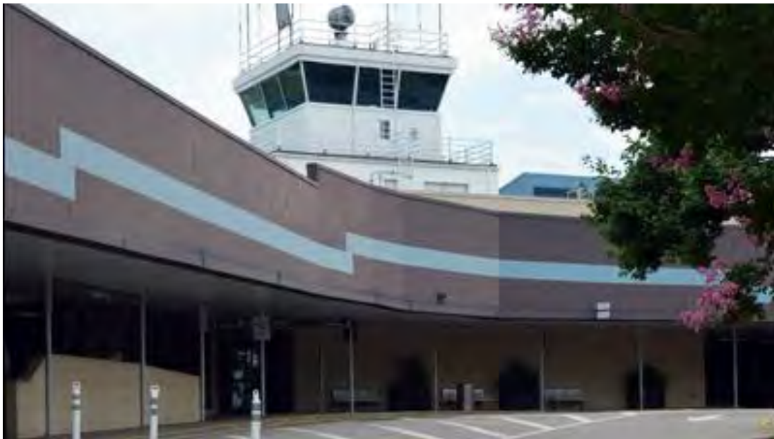
Photo 4. Raleigh-Durham pre-2014 demolition.
