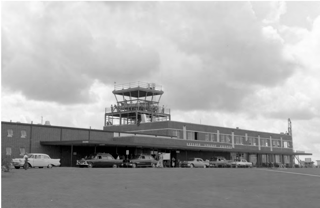
Photo 3. Raleigh-Durham Airport ca. 1955
