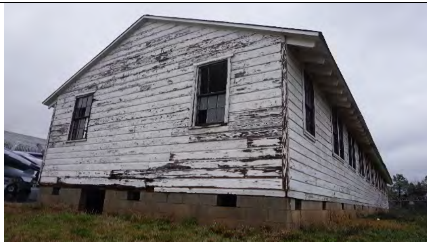
MK3825_ThomasW.FerebeeBuilding,ArmyAirCorpsMorrisFieldBarrac ks_02 20_V.W._04
