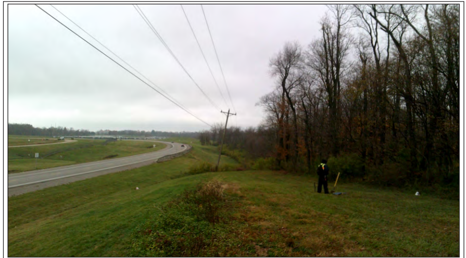
Photo 11. View of Southeastern Disturbed Area Along I-275, Facing South.
