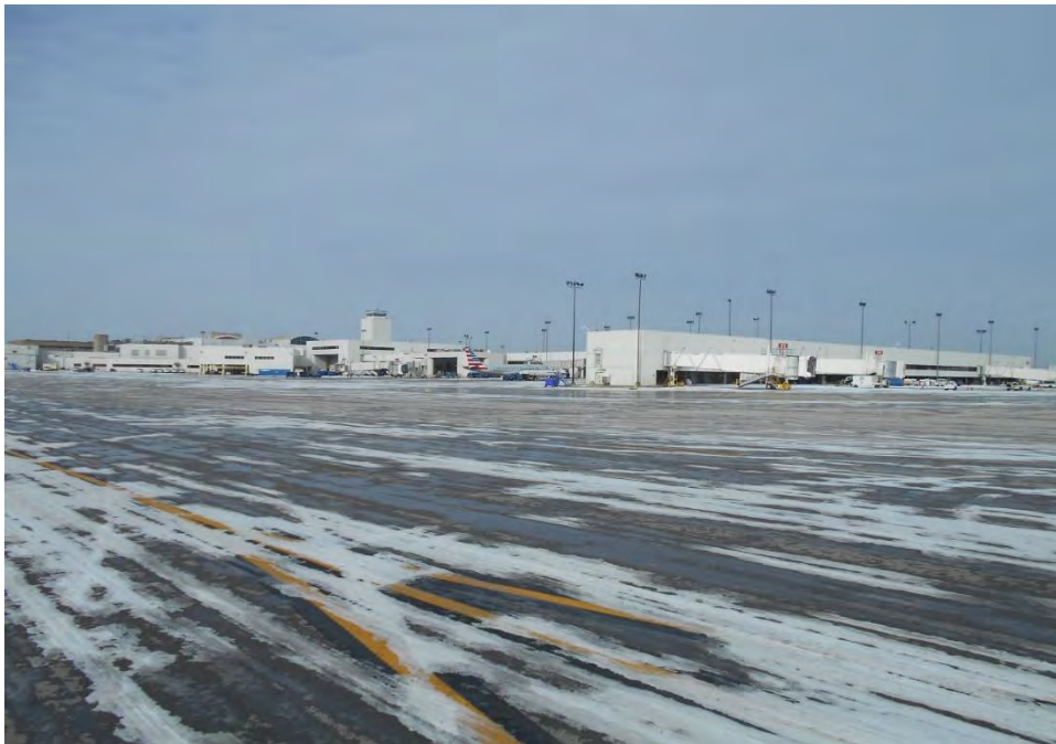
Plate 6. View looking northwest and showing the FRA-10570-12/John Glenn Columbus International Airport Terminal and T-extension.
