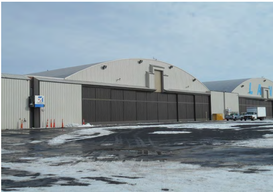
Plate 20. View looking northeast and showing hangar 2 of the FRA-10571-12/Lane Aviation Hangar and Office Facility.
