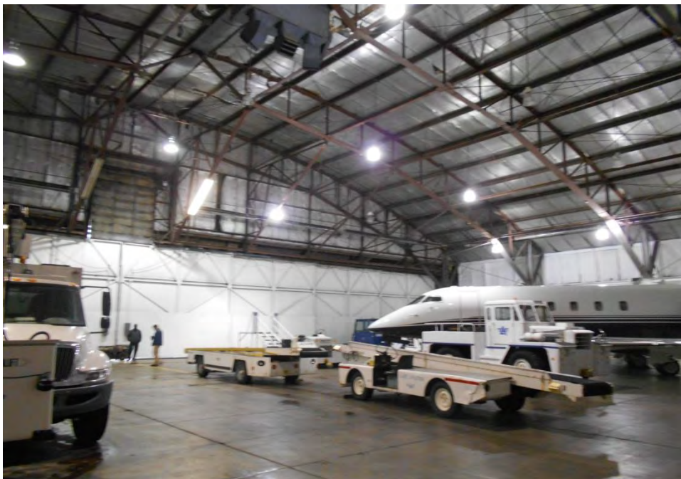
Plate 24. View of interior of hangar 1 of the FRA-10571-12/Lane Aviation Hangar and Office Facility, looking southwest.
