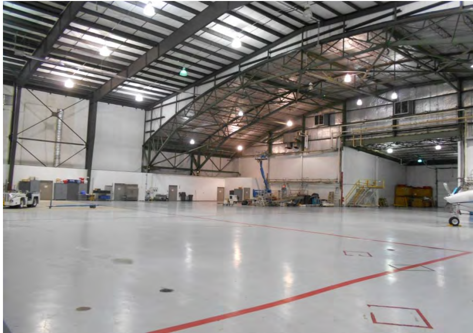
Plate 31. View of interior of hangar 4 of the FRA-10571-12/Lane Aviation Hangar and Office Facility, looking northwest.
