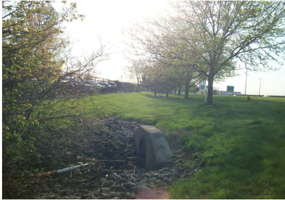
Plate 17. Area 4, culvert at southern end of Mason Run and southwestern corner of former Dollar Rental Car lot, facing east.
