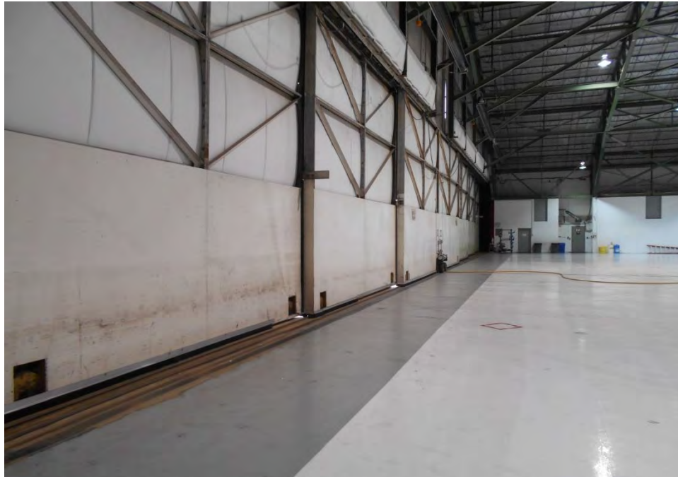
Plate 29. View of the interior side of the doors of hangar 3 of the FRA-10571-12/Lane Aviation Hangar and Office Facility, looking west-southwest.
