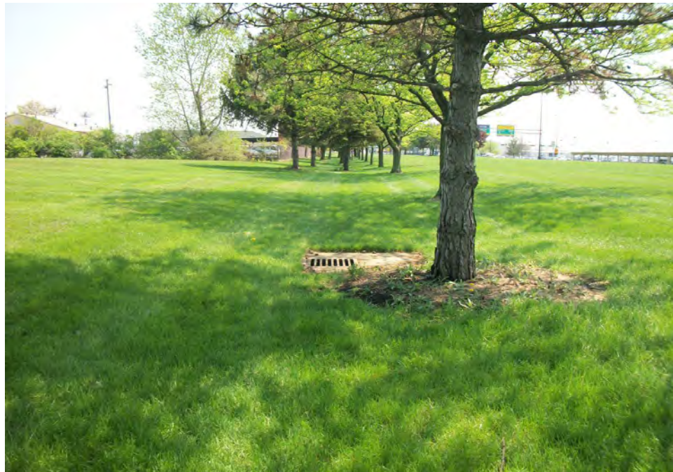
Plate 18. Area 4, storm water drain at base of berm along International Gateway, facing east.
