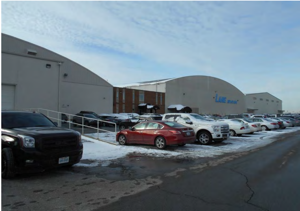
Plate 23. View looking west-southwest and showing the north walls of hangars 4, 5, and 6 of the FRA-10571-12/Lane Aviation Hangar and Office Facility.
