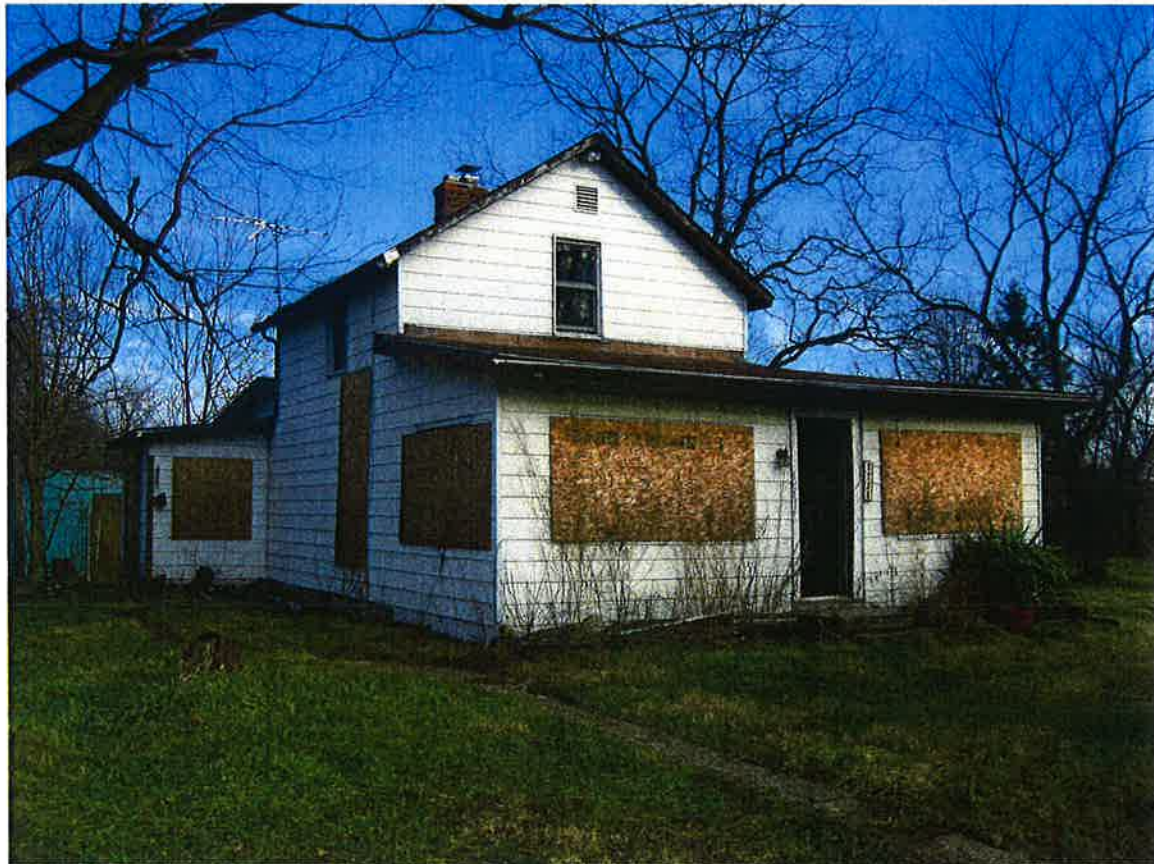
Photo 2: Showing the west and south elevations of the dwelling.
