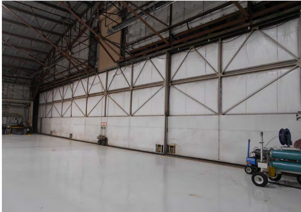
Plate 27. View of the interior side of the doors of hangar 2 of the FRA-10571-12/Lane Aviation Hangar and Office Facility, looking east-southeast.
