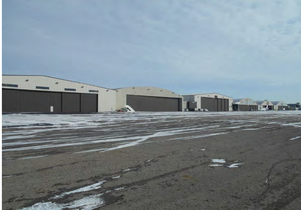
Plate 16. View looking northeast and showing the FRA-10571-12/Lane Aviation Hangar and Office Facility.
