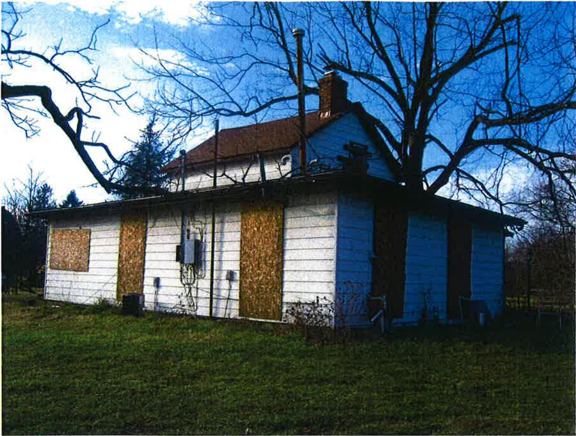
Photo 3: Showing the east and north elevations of the dwelling.
