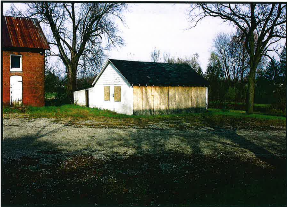
Exhibit 12. Gravel drive and parking area in front of the garage and barn at the Elam Drake house.
