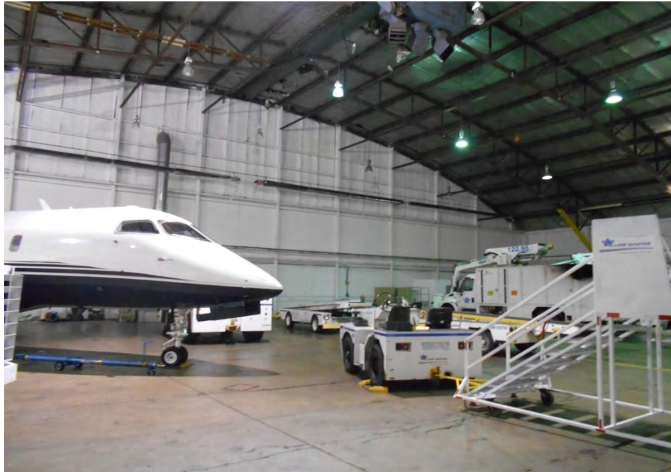
Plate 25. View of interior of hangar 1 of the FRA-10571-12/Lane Aviation Hangar and Office Facility, looking northeast.
