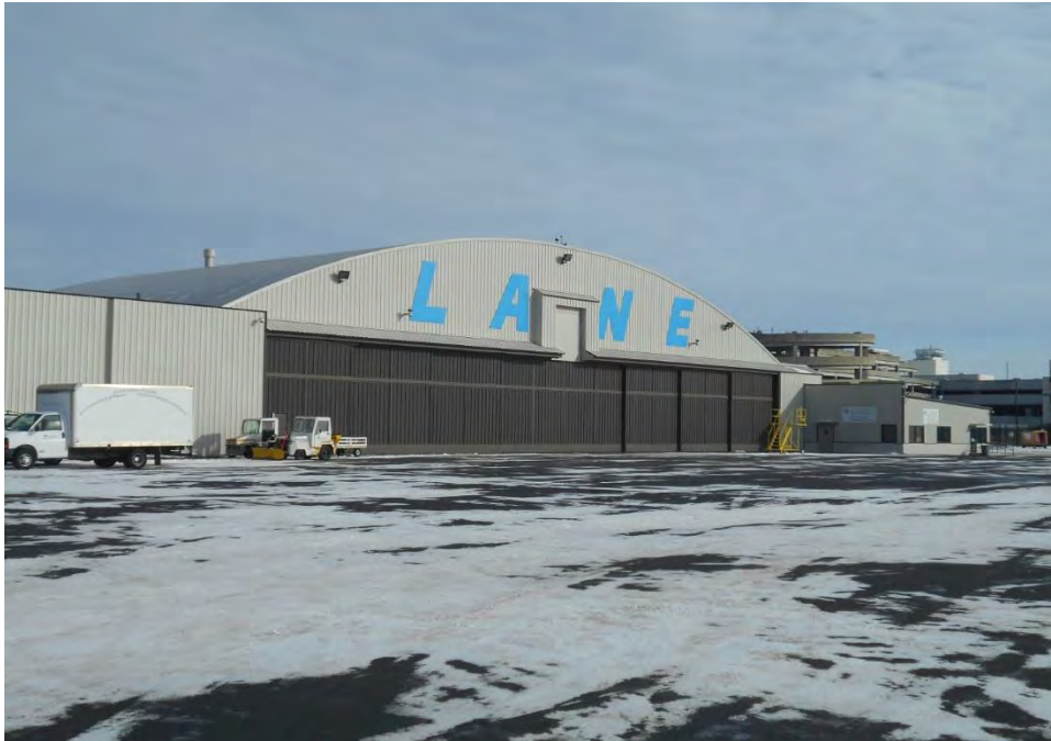
Plate 19. View looking northeast and showing hangar 1 of the FRA-10571-12/Lane Aviation Hangar and Office Facility.
