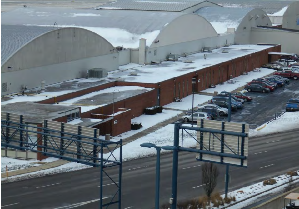
Plate 22. View looking west-southwest and showing the office section of the FRA-10571-12/Lane Aviation Hangar and Office Facility.
