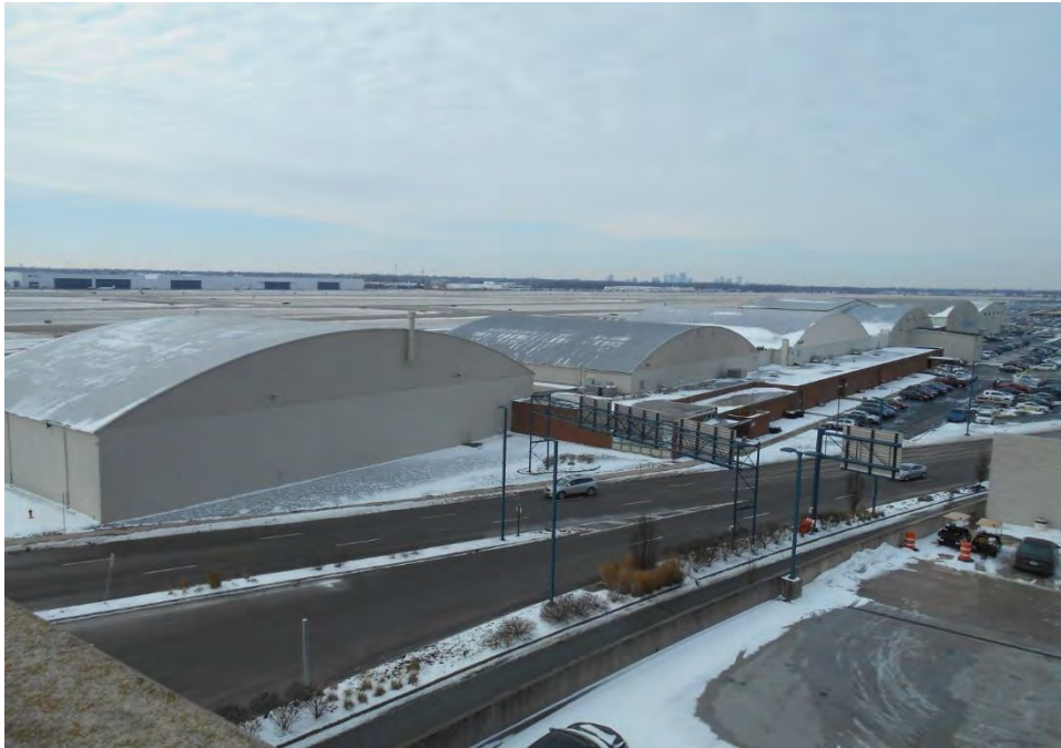
Plate 21. View looking west-southwest and showing the FRA-10571-12/Lane Aviation Hangar and Office Facility.
