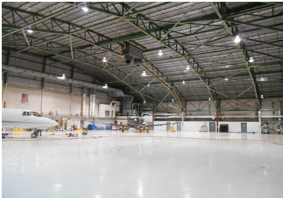
Plate 28. View of interior of hangar 3 of the FRA-10571-12/Lane Aviation Hangar and Office Facility, looking northeast.
