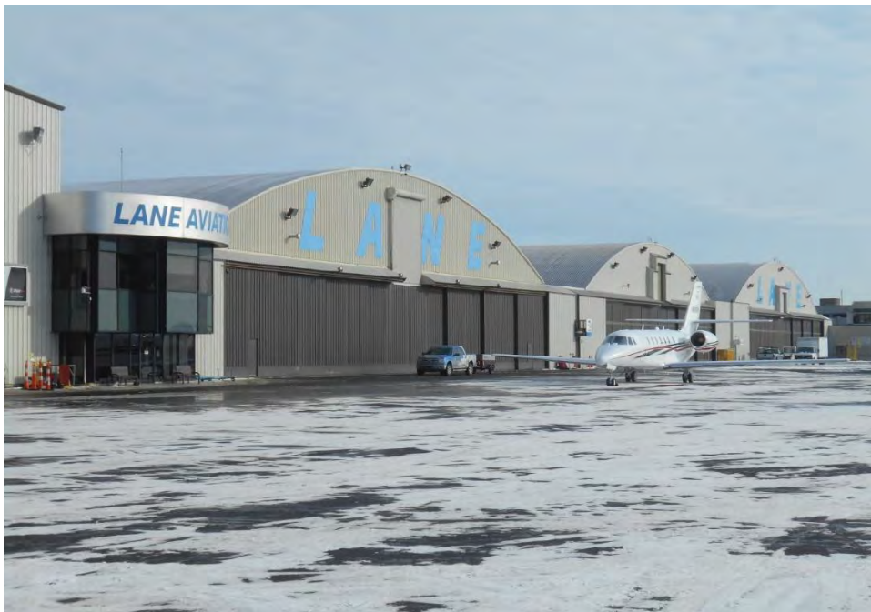
Plate 18. View looking northeast and showing hangars 1, 2, and 3 and the entrance to the main lobby of the FRA-10571-12/Lane Aviation Hangar and Office Facility.
