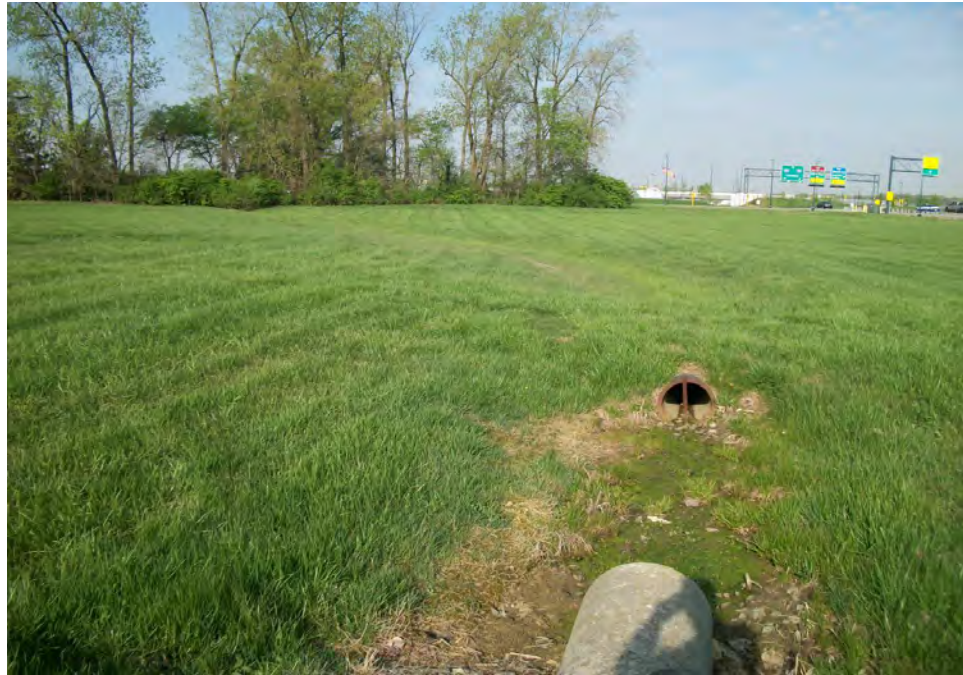
Plate 11. Area 2, open drainage ditch, facing west.
