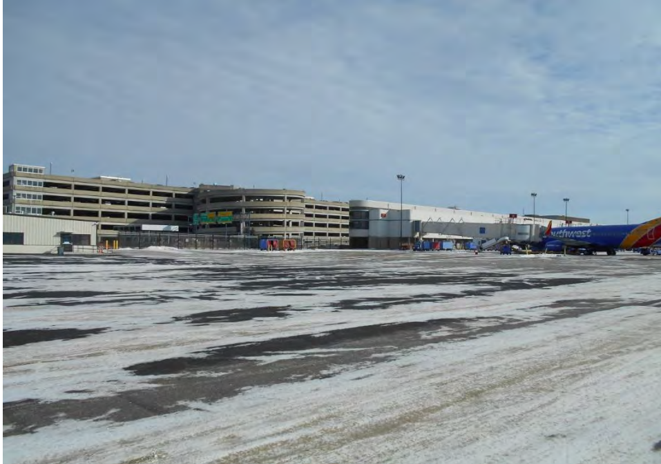
Plate 7. View looking northeast toward the FRA-10570-12/John Glenn Columbus International Airport Terminal and showing a portion of the 2000 parking garage and 1989 Concourse A addition.
