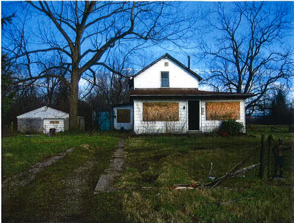
Photo 1: Showing the dwelling at 2743 Ole Country Lane.
