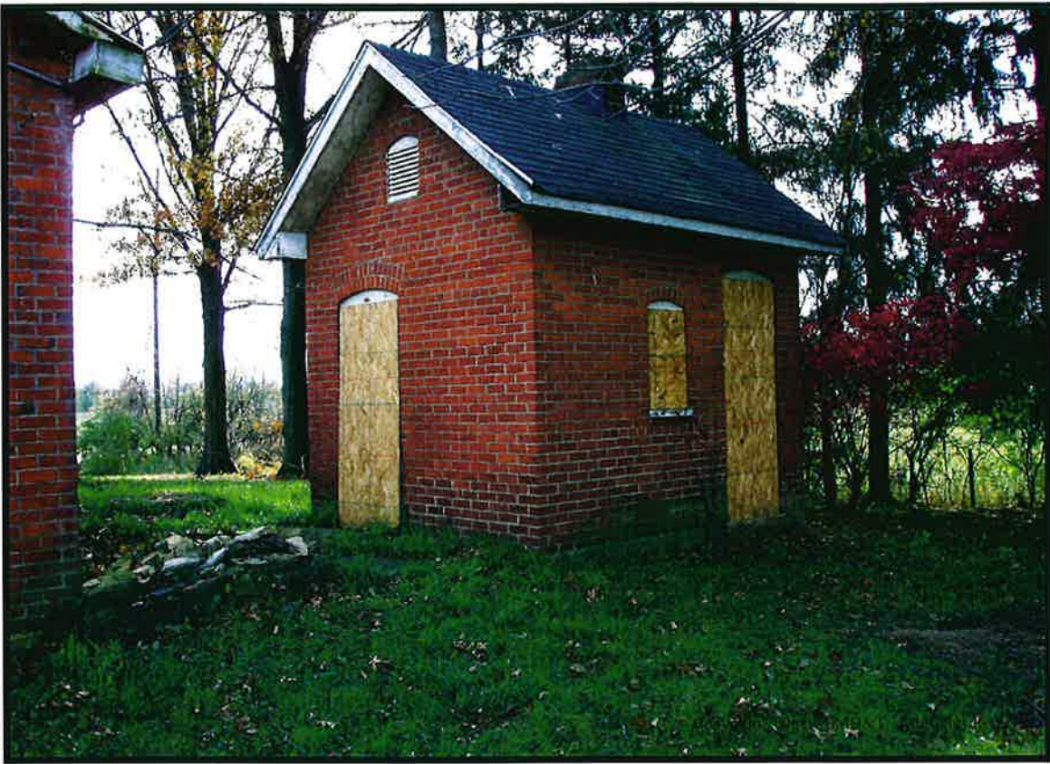
Exhibit 13. Smokehouse located northwest of the Elam Drake house.
