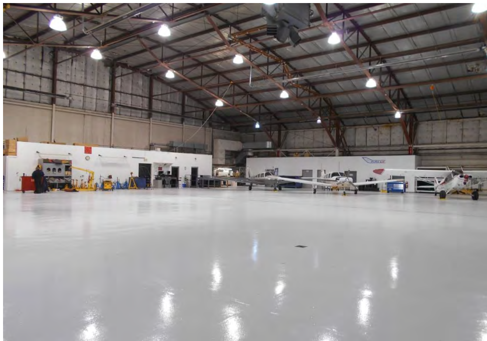
Plate 26. View of interior of hangar 2 of the FRA-10571-12/Lane Aviation Hangar and Office Facility, looking northeast.
