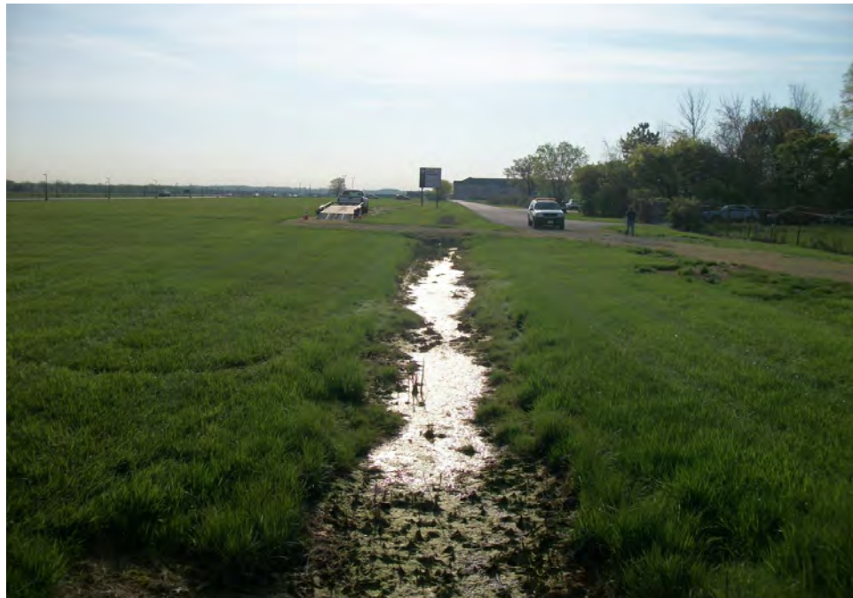
Plate 14. Area 3, open drainage ditch, facing east.
