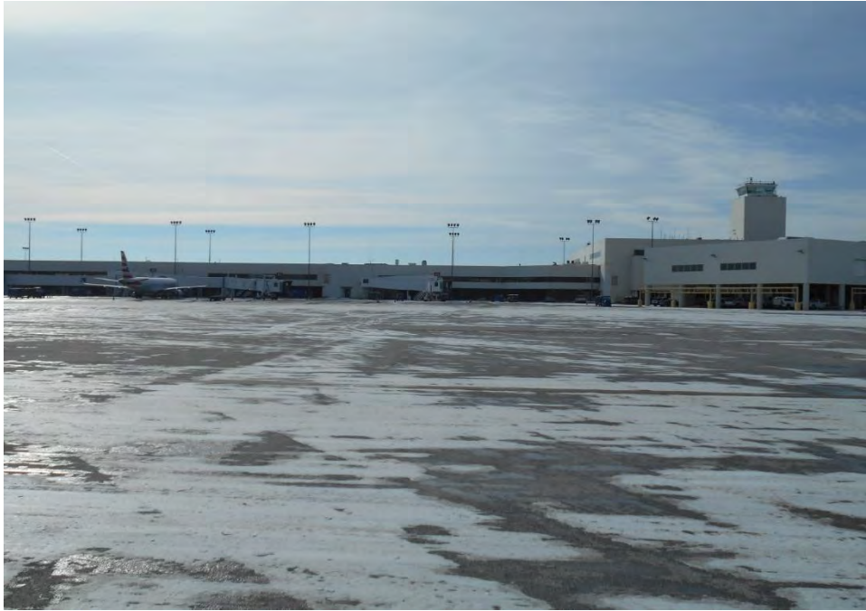
Plate 5. View looking south toward the FRA-10570-12/John Glenn Columbus International Airport Terminal and showing a portion of what remains visible of the 1958 terminal and “passenger loading pier.”
