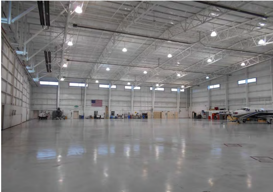
Plate 33. View of interior of hangar 6 of the FRA-10571-12/Lane Aviation Hangar and Office Facility, looking northwest.
