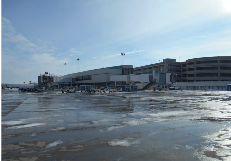
Plate 10. View looking southeast toward the FRA-10570-12/John Glenn Columbus International Airport Terminal and showing a portion of the 2000 parking garage and Concourse C additions.
